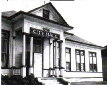
The picture above is of this wonderful old building, page 88, Jim Felton's book "Newport Beach, the First Century," available at the Balboa Library. (Page 3)
